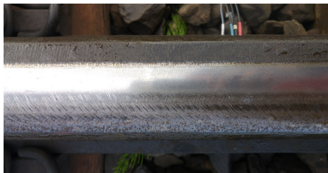
Fig. 1 – A head checking defect Source: own elaboration
