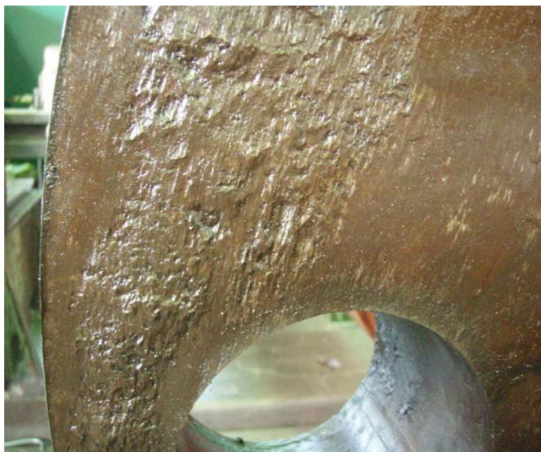
Fig.4. An example of failure of the shaft collars and fitted bolt holes in the propulsion shaft [4].
