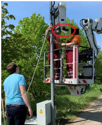
Figure 2. Hanging measurement module of an intelligent road sign in Lezno, Poland. At the bottom of the suspended box, marked with a red ellipse, microphone and camera is seen.
