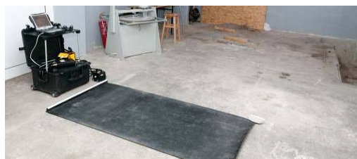
Fig. 4. Ground floor structure during GPR surveys
