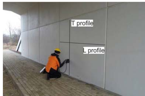
Fig. 8. Abutment of railway viaduct
