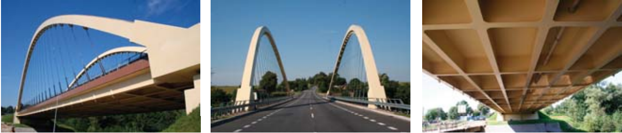
Fig. 3. Construction of the bridge in Poganice
