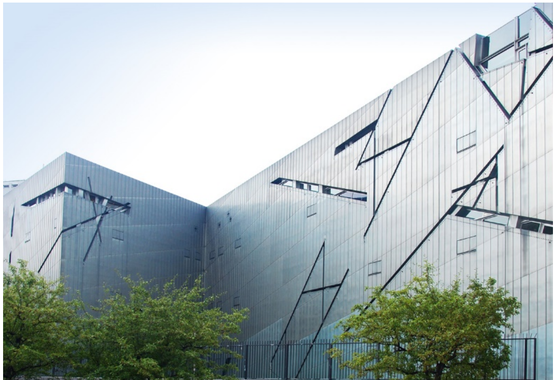
Fig. 3. The Jewish Museum façade covered with zinc panels cut by irregularly shaped glazing. Source: photo J. Badach
