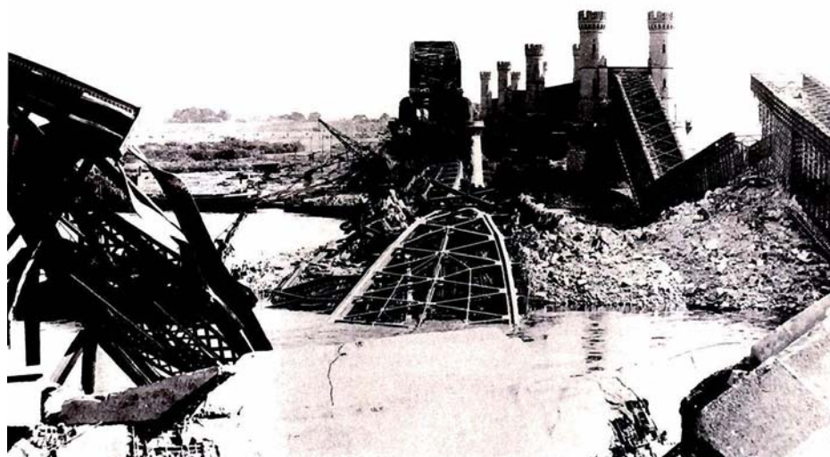
Fig. 3. War damages of bridges in 1938
