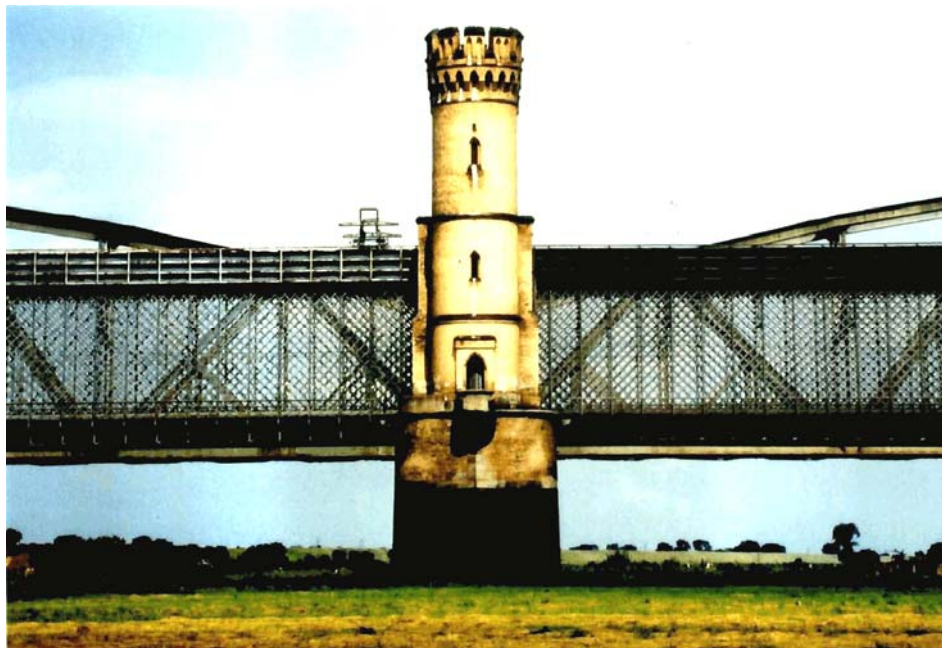
Fig. 5. Side view of bridges
