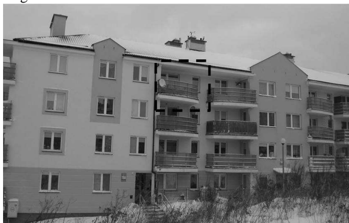
Fig. 1. Reference building in Gdańsk with the selected spot measurements (Foto by: R.Antczak-Jarząbska)
