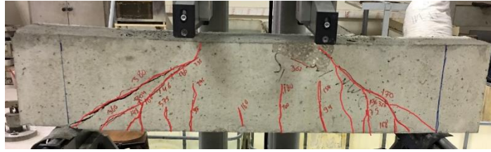
Fig.9: Beam (B1) at failure
