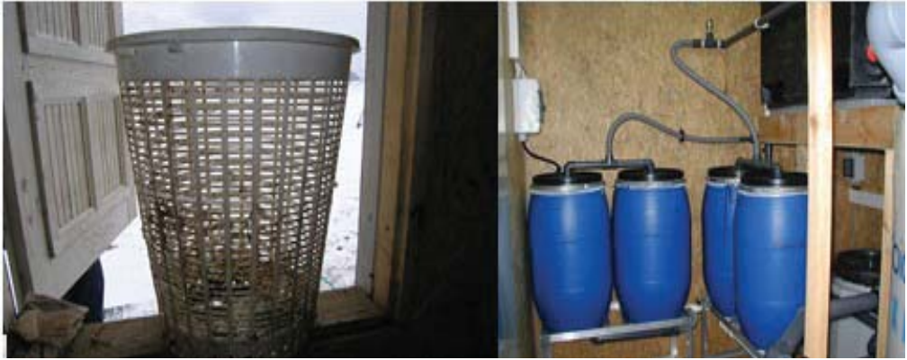
Fig. 3. Sludge processing at the Biovac® wastewater treatment plant [10]
