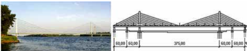
Fig. 17. Solidarity Bridge in Plock, Poland (2002) (photo: wikipedia)
