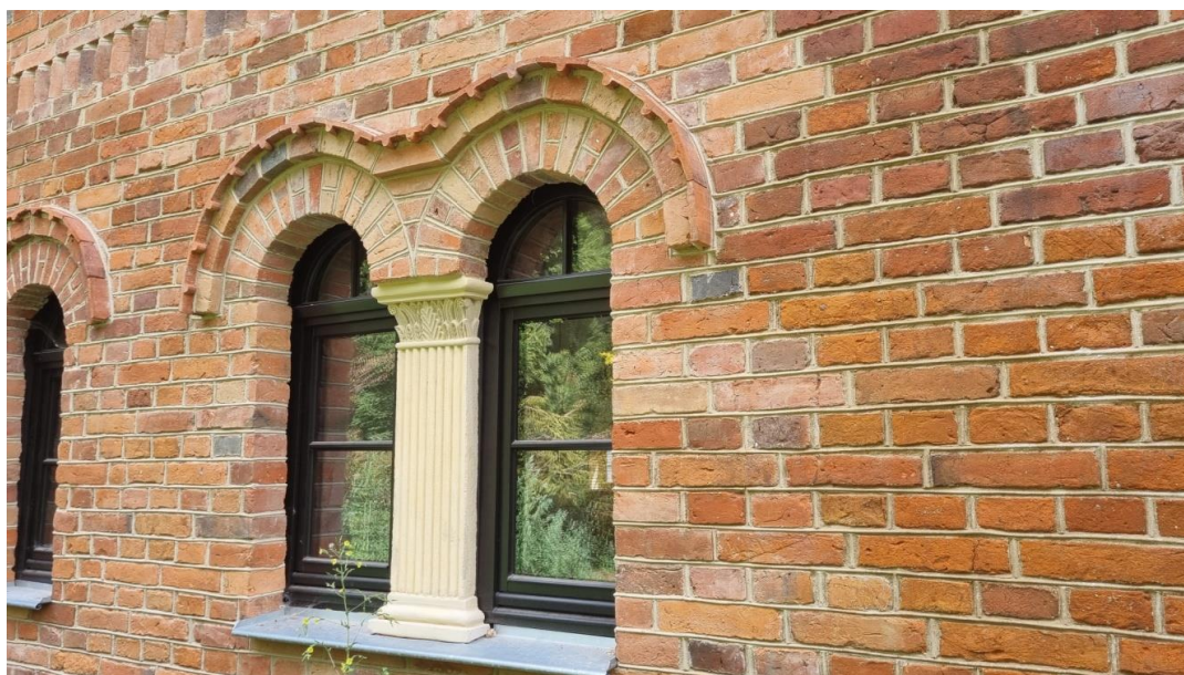
Fig. 19. Revitalization of historic solid ceramic brick wall using contemporary brick and ceramic tile and limestone details (photo: Maciej Niedostatkiwicz)
