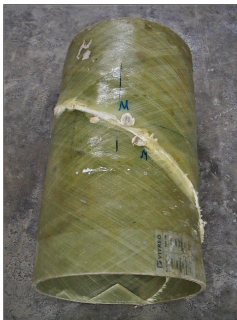
Fig. 9. Destroyed composite coating
