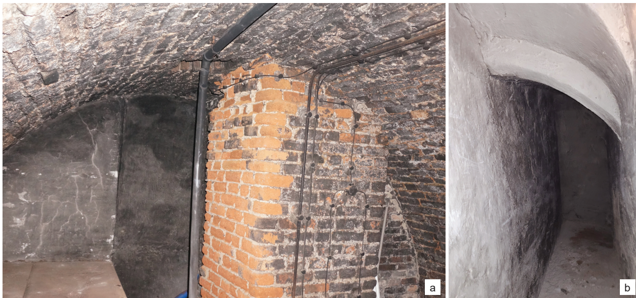
Fig. 6. Underground parts connected with the chapel at St. Joseph's Church in Gdańsk: a) a view of the interior of the crypt under the eastern part of the chapel towards the south, b) a fragment of the present corridor connecting the former crypt with the chancel (photo by A. Piwek)
