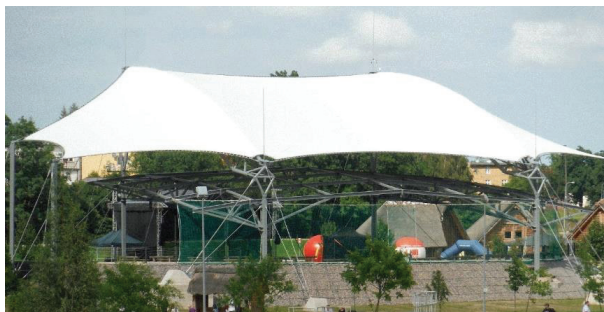
Fig. 1. Membrane hanging roof in Pruszcz Gdanski
