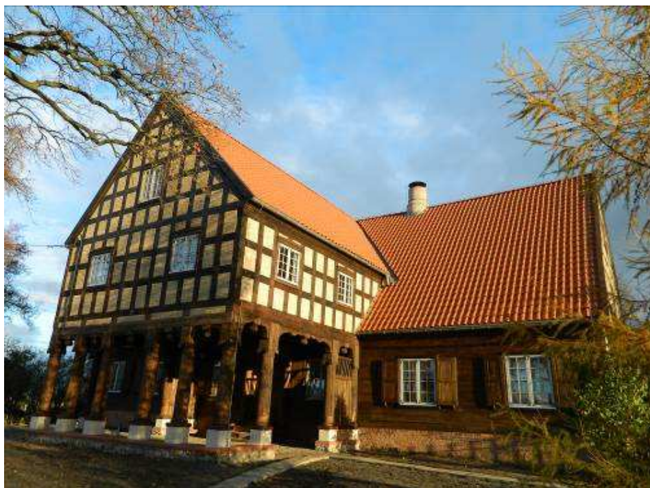
Fig. 2. Arcade house in Marynowy upon completion of building-conservation works
