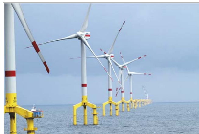
Fig. 1. Tripile-type platforms – project BARD offshore 1 – Germany. Approximate depth of water area 40m [www.windpoweroffshore.com, www.hadel.net]
