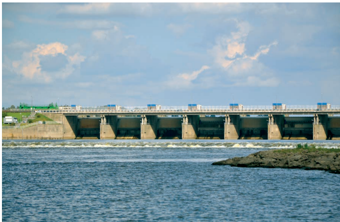
Photo 6. The Włocławek barrage, view from the lower water, photo: P. Jerzyło
