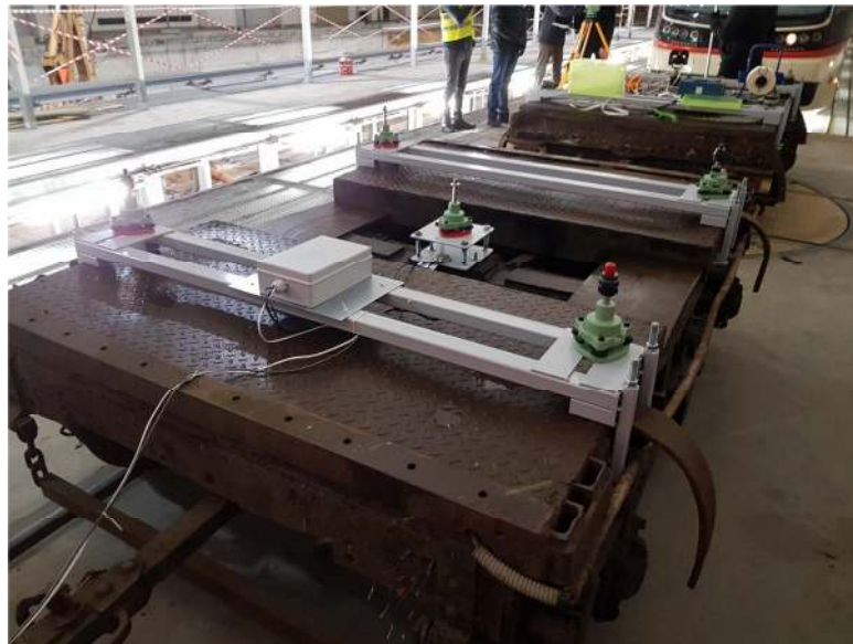
8. Assembly of racks (with tribrachs) on measuring bogies - Tram Depot Wrzeszcz
