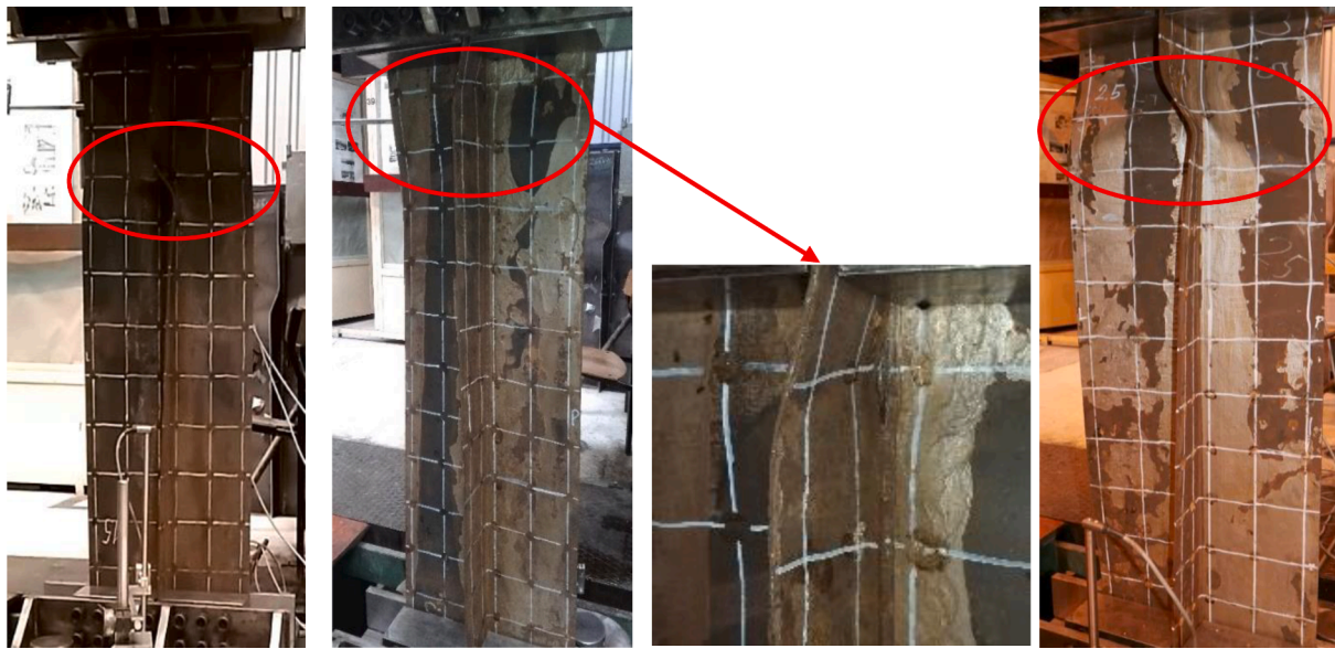
Fig. 9. Post-collapse shapes for 5 mm specimens with degradation level of 7% (left), 14% (mid) and 21% (right).
