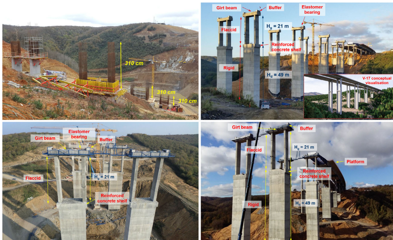
FIGURE 24 Photos from the application of the new DDC2 algorithm on the Northern Marmara Highway construction site
