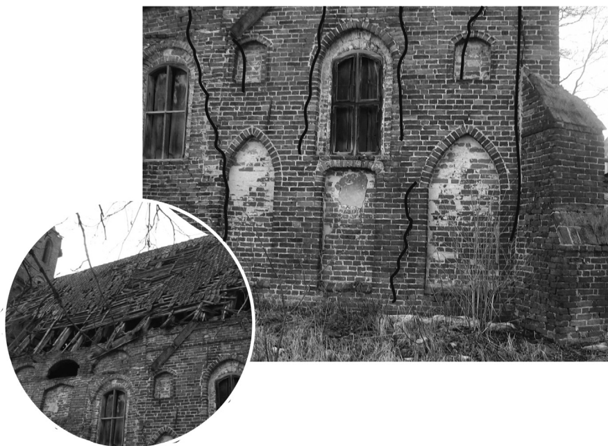
Fig. 5. View of the south wall and roof over the wall.
