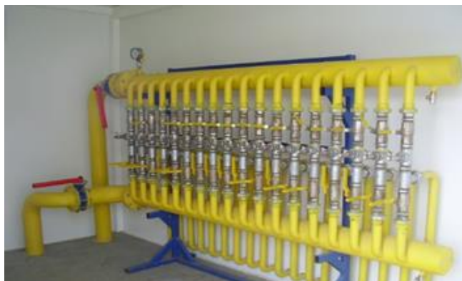
Fig. 3. Connection of gas wells to main pipelines (13)
