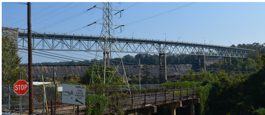
Figure 2. Fitzpatrick Bridge side view.
