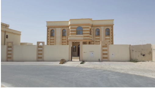
Figure 10. Acquisition and cataloging department offices.
