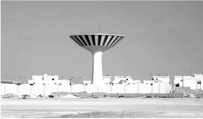
Fig. 3. Water Storage Tank in Al Ghanem area
