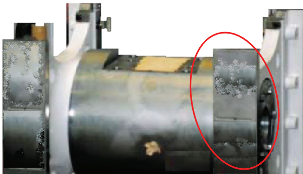
Fig. 9. View of excessive friction and corrosion wear, accompanied by local deep losses of material in the surface layer of the crosshead shoes 3 (Fig. 5) [36]
