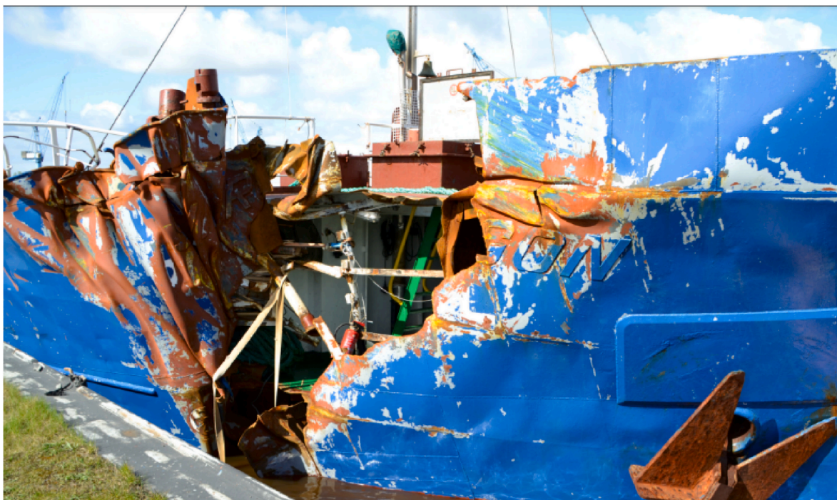
Fig. 2. Collision damage of the ship Petra L. (LOA = 74m) on the Gode Wind 1 offshore wind farm (monopiles D = 6\text{m} , 6 MW) (Mandra, 2023).
