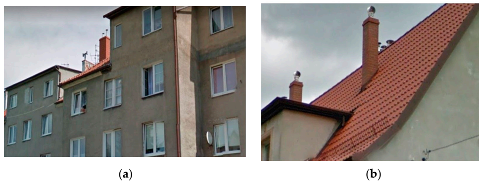
Figure 21. Multi-family housing in Gdańsk: (a) traditional chimney cap and (b) rotary type chimney cap.
