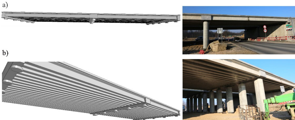
Fig. 3. The comparison of the computational model and real structure, a) side view, b) bottom view.
