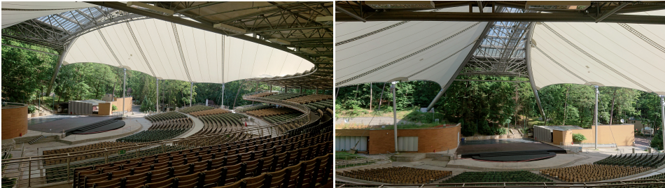
Fig. 1. The Forest Opera membrane hanging roof in Sopot, Poland – co-designed by the authors
