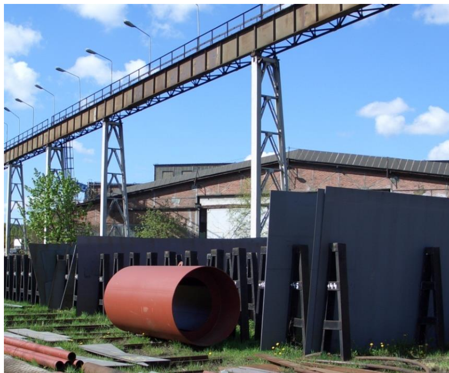
Figure 2. Gdansk Shipyard, metal sheets warehouse for shipbuilding on the site of the future European Solidarity Centre (ECS) building (photo by Wojciech Targowski).
