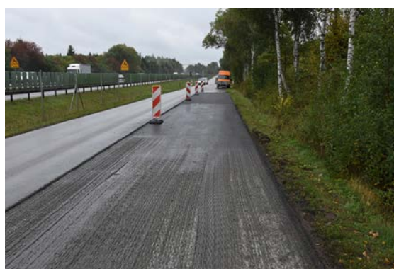
Figure 17. New binder course after surface milling.
