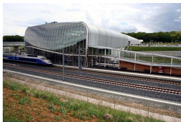
Figure 2. Belfort-Montbéliard TGV (D.Zaluski). Distinctive form of the tube made of laminated wood covered with galvanized steel helps to reduced energy consumption.
