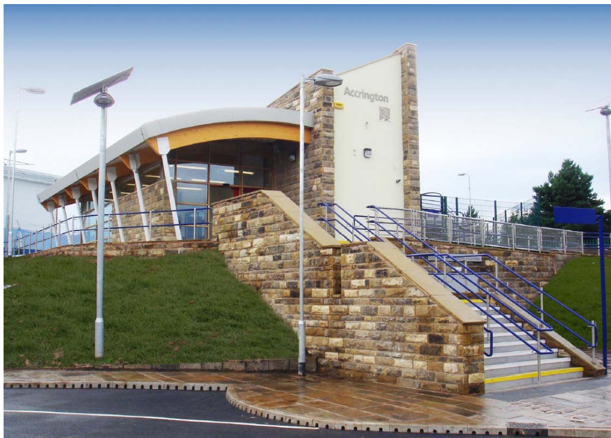
Figure 3. Accrington Eco Railway Station (SBS ARCHITECTS LTD. 2010 from [9]). Application of a local stone integrated the building with architectural heritage of the historical part of the city and helped to reduce transportation needs in terms of range and costs
