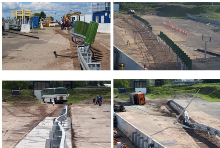
Fig. 1. Photographic documentation of the crash tests conducted for the ROSE project
