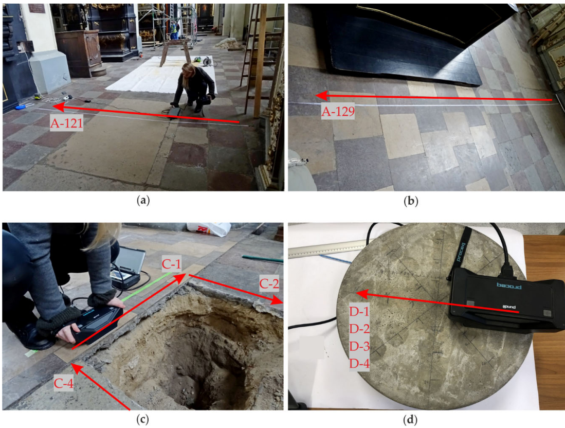
Figure 8. Ultrasonic measurements: (a,b) along traces A-121 and A-129 in the south aisle; (c) along edges of the trial pit; (d) along circular slabs.
