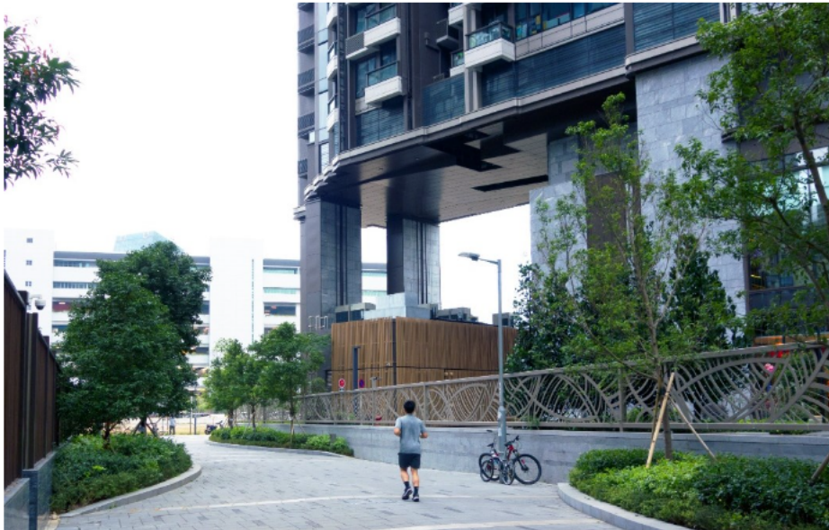
Fig. 4. The Kai Tak Development in Hong Kong – a project, in which the design solutions for urban ventilation enhancement were applied, including open ground floor plans and building voids to facilitate air flow between buildings. Photo: Joanna Badach.
