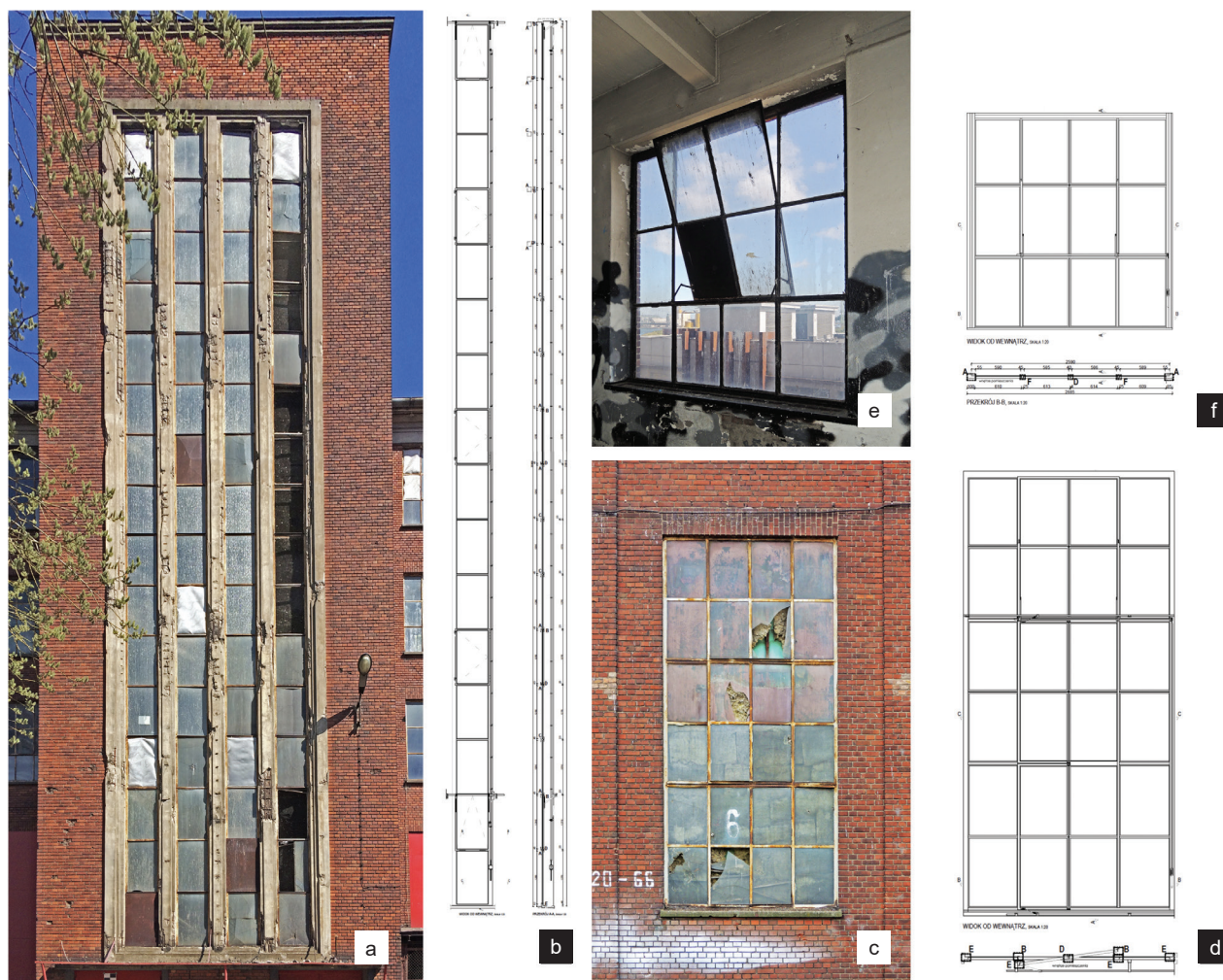
Fig. 9. Variety of metal windows covered by the detailed examination of the Main Warehouse (89A), so-called the U-Boat Hall. All industrial windows were of a type so-called “complex” windows, made of steel, rolled elements, of the standing or lying type, with fixed or tiltable sections, 2018–2019: a, b) staircase avant-corps (TYPE 4 window) in the southern elevation – a sixteen-row, single-section window, dimensions: width 95 cm, height 2081 cm; five single-deck opening wings, c, d) ground floor (TYPE 2 window) – a six-row, four-section window, dimensions: 260 cm, height 551 cm; three four-quarters wings in the central part with hinged openings, e, f) window of upper floors (TYPE 1 window) – a three-row, four-section window, dimensions: width 268 cm, height 287 cm; four-quarters vertically tilting section that opens vertically (source: [22])
