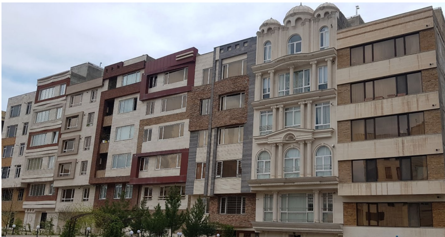
Fig. 1 Adjacent buildings in Tehran with different floors and base levels without separation distance
