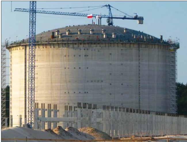
Fig. 1. View of the tank during its construction
