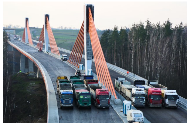
Fig. 5. Full ballast loading during U45 setting.
