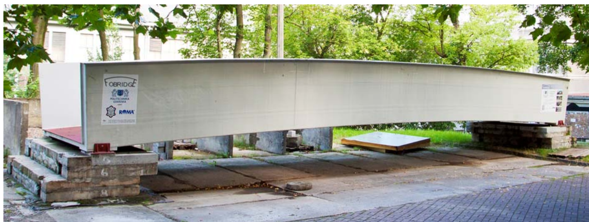
Figure 1. U-bridge located on the Gdańsk Technical University campus
