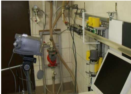
Figure 3. A general view of the measurement section of the installation.
