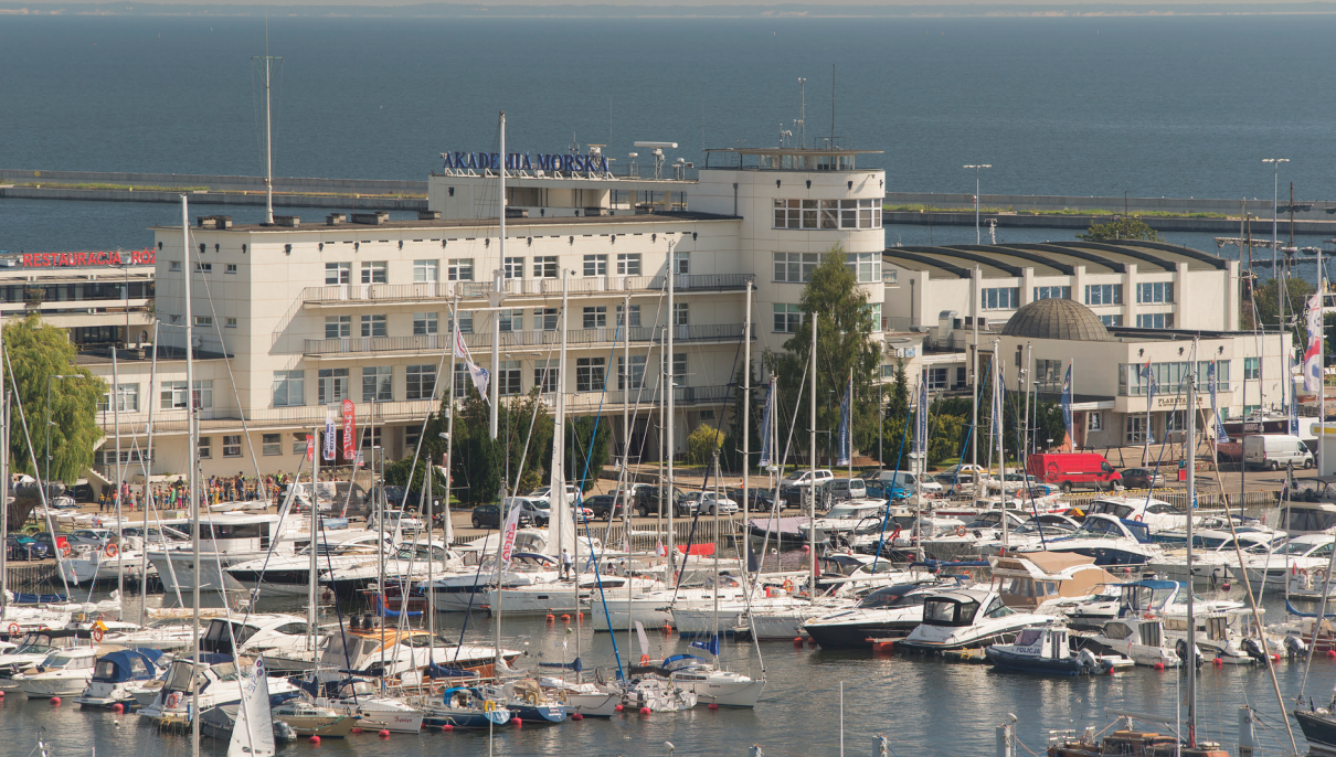
Fig. 2: Gdynia Maritime Academy on the South Pier (built 1938-1939), 2017
