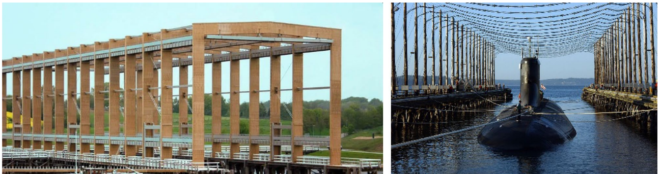
Figure 1. Earth's magnetic field simulators 20,21 .
