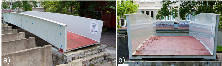
Fig. 8. Composite footbridge designed within the FOBRIDGE project in Gdańsk, Poland
