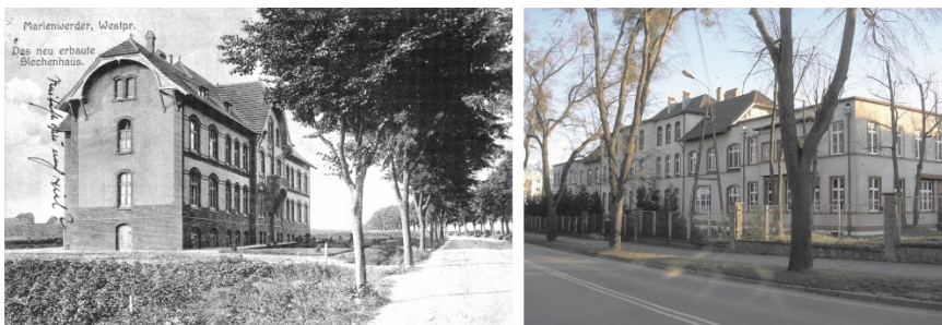
Figure 5: County hospital in Kwidzyn, the state dating back to the beginning of XX century (left) and present (right). Example of a ever-growing hospital, with many extensions.
