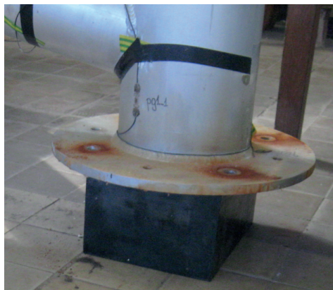
Fig. 2. Conditions of tripod foundation on rubber blocks.
