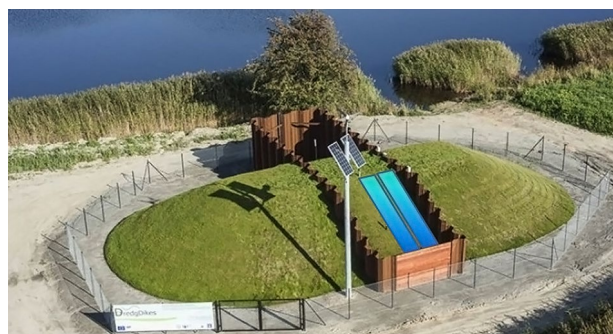
Fig. 3. Gdansk research dike with test section and location of flume 1 (right) and flume 2 (left)
