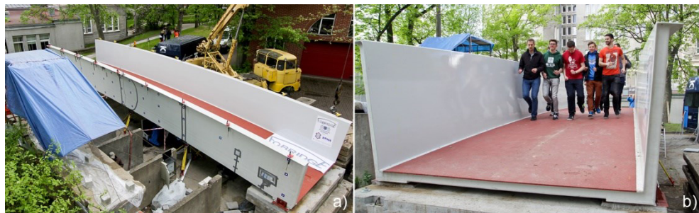
Fig. 8. GFRP footbridge constructed within Fobridge project.
